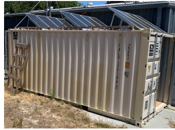
Fig. 7. Microgrid enclosure and PV arrays
